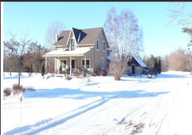
Front house view w/original ice house at side
